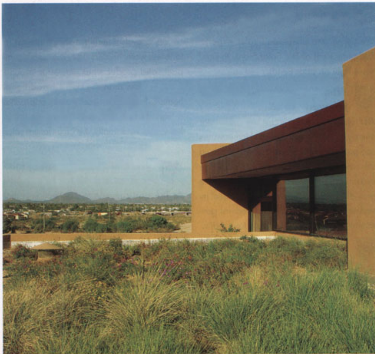
Second-floor windows peer out onto a landscaped area rather than a bare roof.
